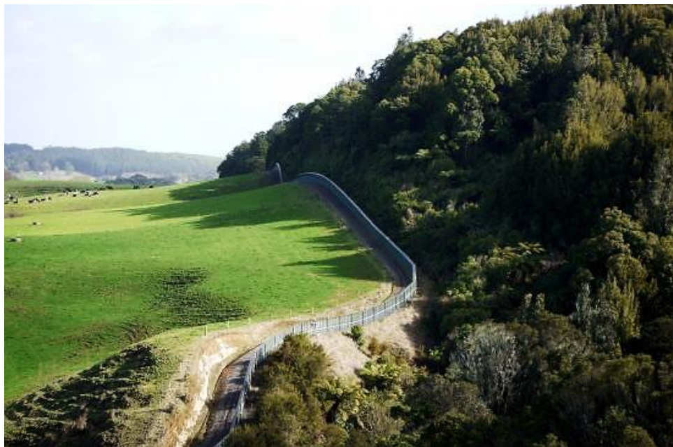
Image caption: A 47-kilometre-long pest-exclusion fence encircles Sanctuary Mountain Maungatautari, creating a secure ecological haven completely isolated from the surrounding agricultural landscape of Pukeatua. This monumental barrier is one of the largest of its kind in the
